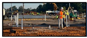
Plumbing for the lobby area has been run and stubbed up in preparation for the slab on grade in that location
