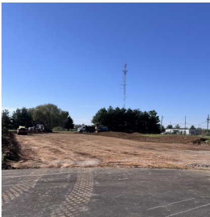
Construction begins on additional parking lot
